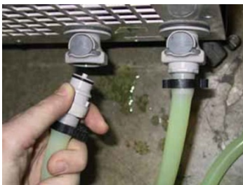
Figure 22: Remove Exchanger Tubing Connection
