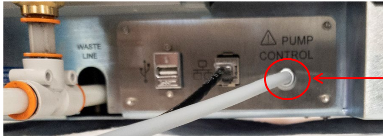
Figure 5: Connect Pump Control
